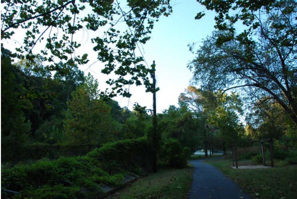
Figure 4 View along the Holmes run trail - collapsed court fence on the left
